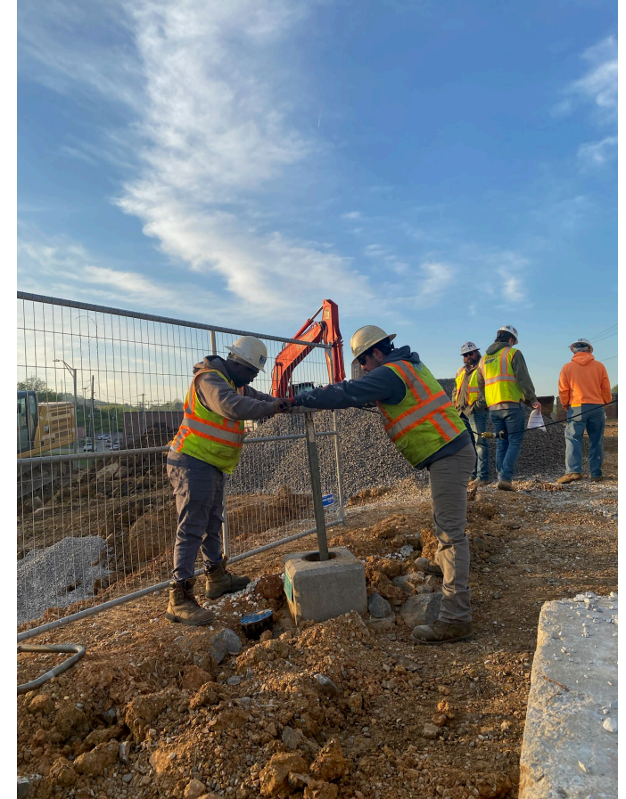
Two KUB UGC employees operate an intermediate valve
