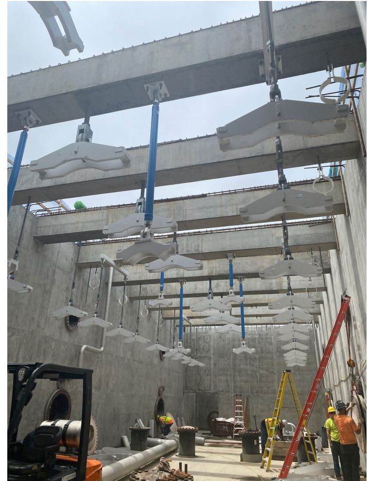
Pipe hangers, piping, and other construction activities occurring within the filter pipe gallery
