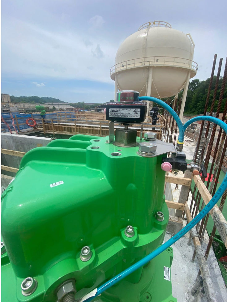
Washwater tank and a filter control valve
