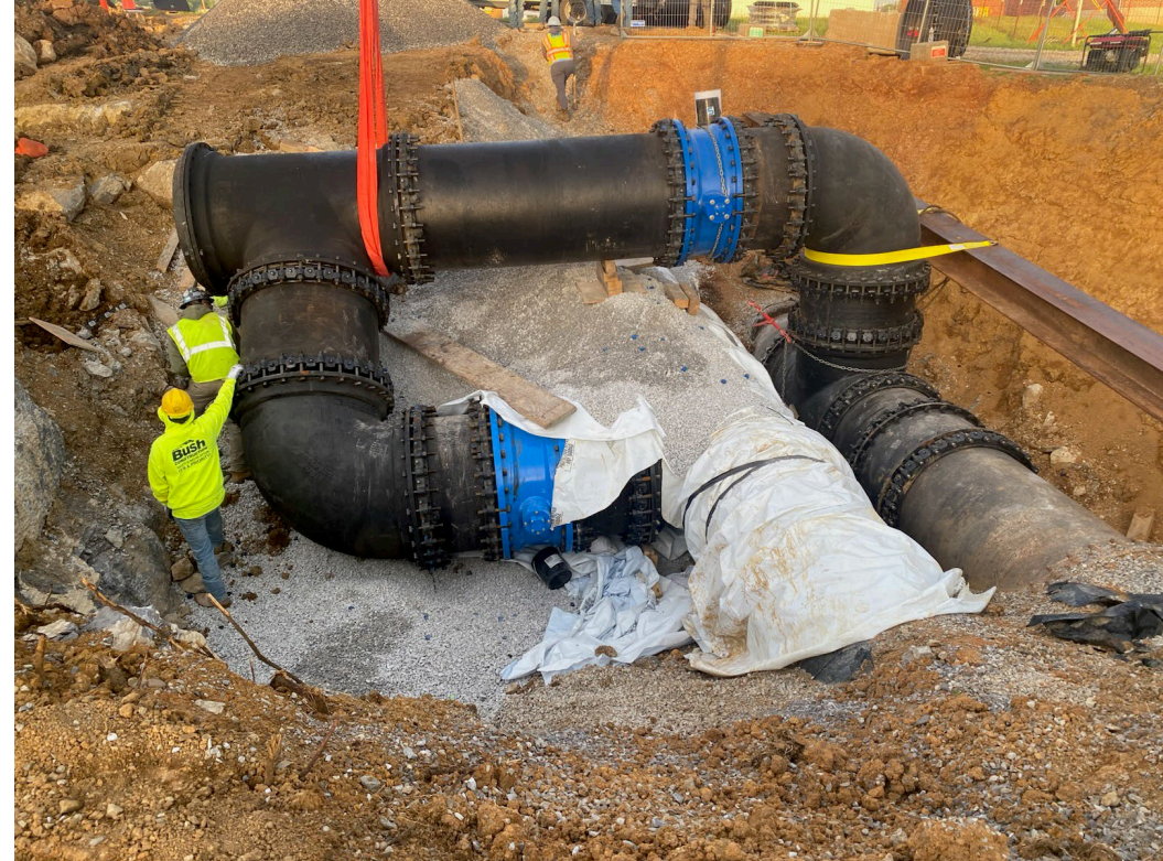
Tie-ins to existing MBW intermediate lines
